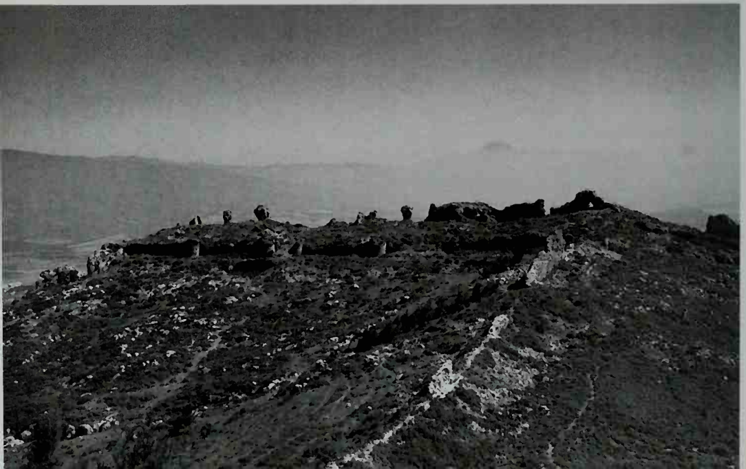
19. High above the city, atop Mount Silpius, stood the citadel of Antioch (BELOW). Built to withstand attack both from outside the city and from within, no force could claim true dominion of Antioch without possession of this fortress.
