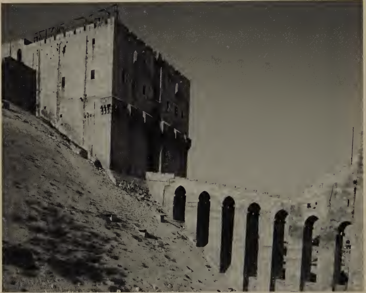
14. Entrance gate-tower and bridge to the citadel of Aleppo, built in the twelfth and early thirteenth centuries, in part by the dynasty of Salah al-Din (Saladin), one of the many remarkable fortifications built at the time of the Crusades.
