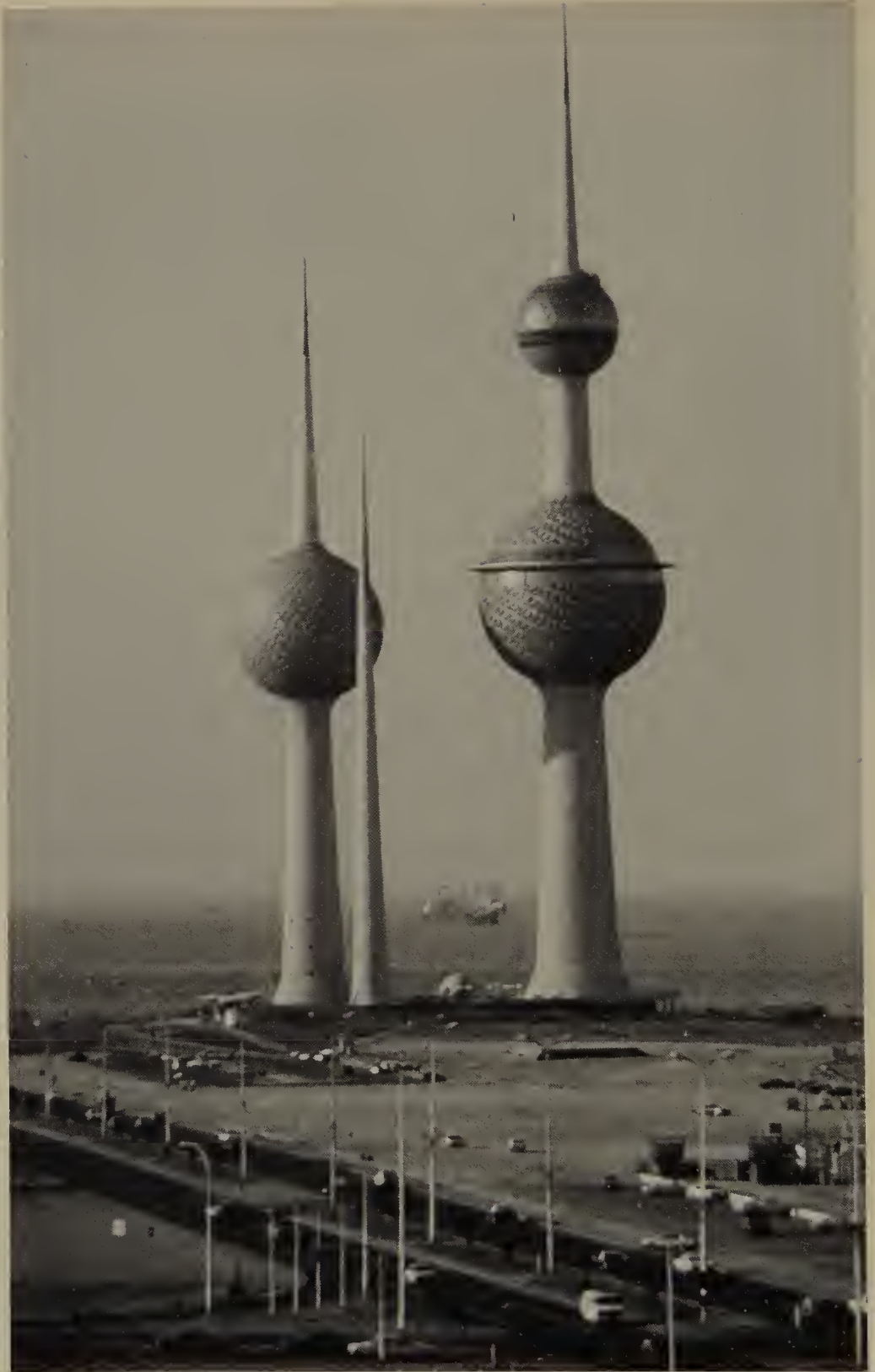
36. Kuwait Water Towers in Kuwait City, which won the Aga Khan Prize for Innovation in 1980. They represent the kind of bold modernistic architecture that the new prosperity of modern Arab oil states has made possible.
