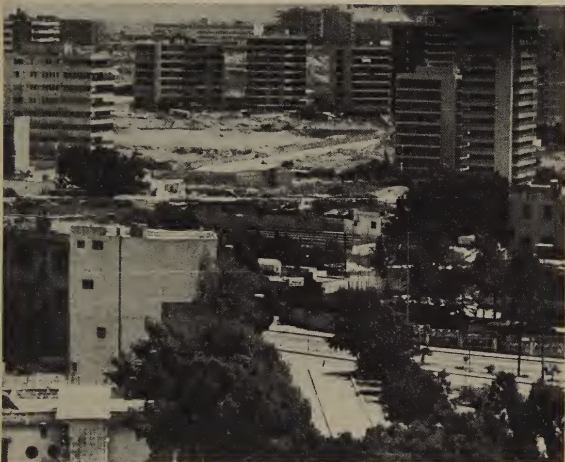
32. Residential buildings in modern Beirut. With the growth of Beirut as a financial center after the Second World War, large numbers of luxury flats were built, not only to accommodate the Lebanese but also to house foreigners from Europe and other parts of the Arab world; many became empty shells in the Lebanese civil war (see pp. 430-3).
