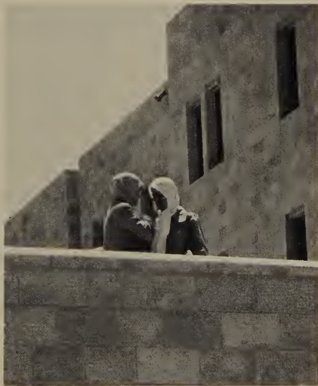
38. The Najah National University, Nablus, on the West Bank, in which this postmodernism appears in a more stark form, recalling Arab public buildings of the Levant in the prewar period.
