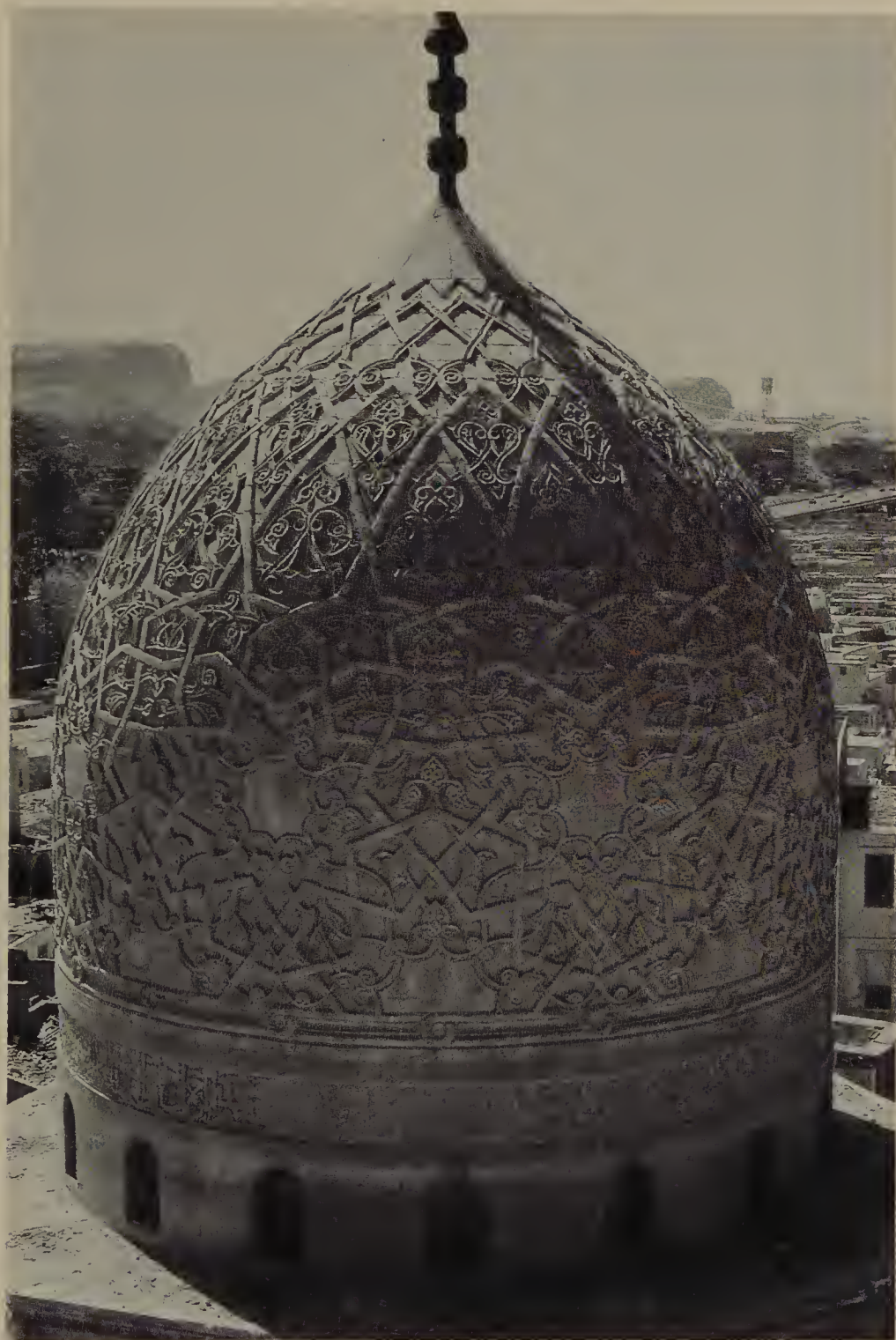
15. Dome of the mausoleum of the Mamluk sultan Qaytbay in Cairo, built in 1474. Carved masonry domes, with extraordinary integration of Arabesque and geometric ornament, were the specialty of Cairene builders. Like many funerary complexes of Mamluk rulers, it included a permanently endowed school.
